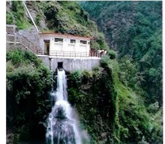
Small Hydro Power Plant
