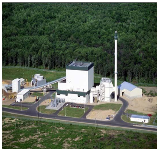
37.5 MW Plainfield Biomass Power Plant, Connecticut New England, USA.
